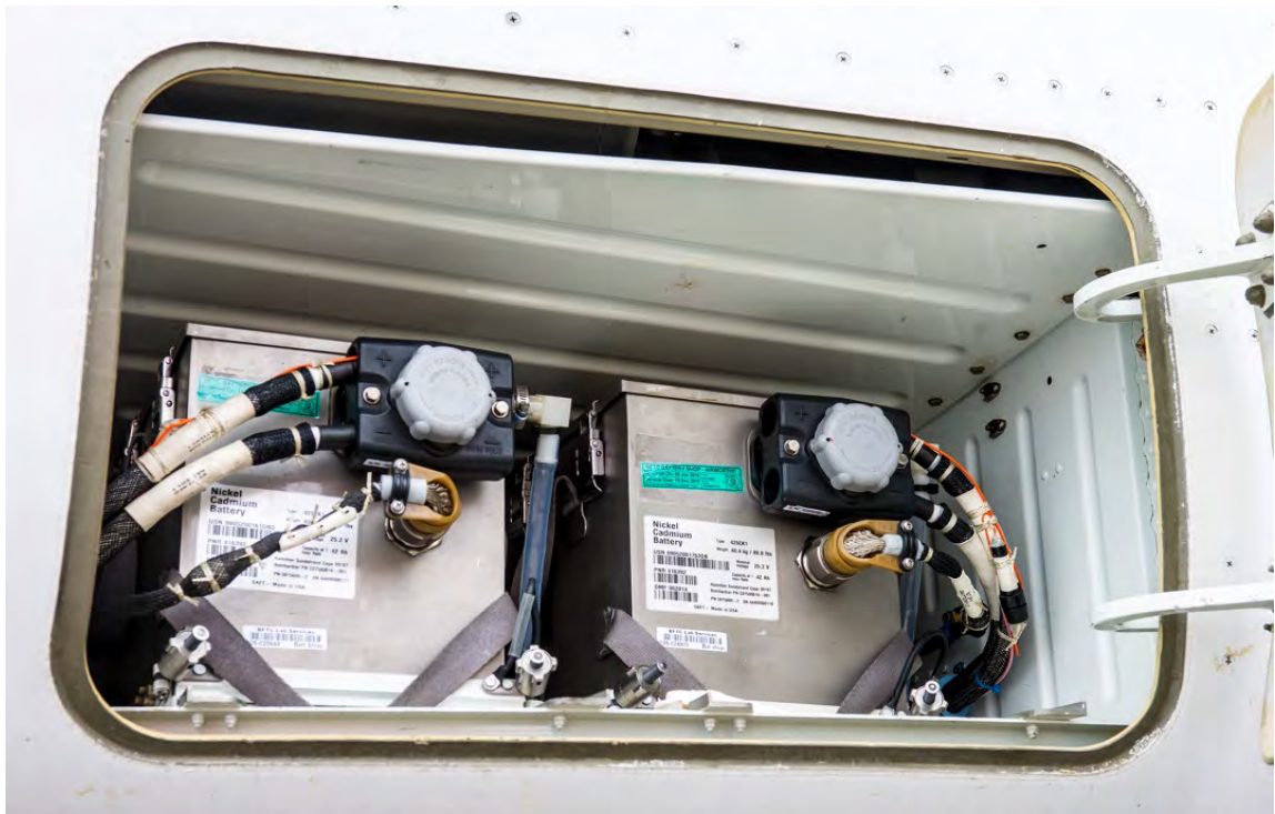
Figure 2.1. : compartiment des batteries (photo © Pierre Gillard).
